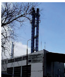
District Heating Plant of EMPEC Ustka Ltd.
